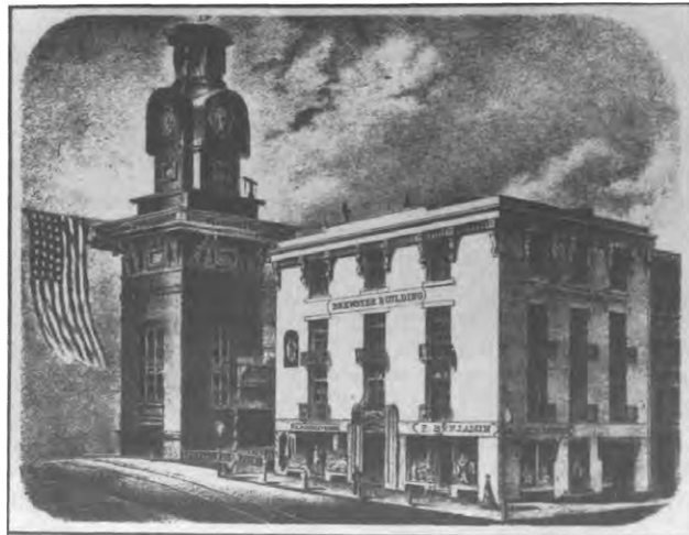
Brewster Building, southeast corner of State and Chapel Streets, New Haven. First floor rooms served as synagogue 1846–1856
