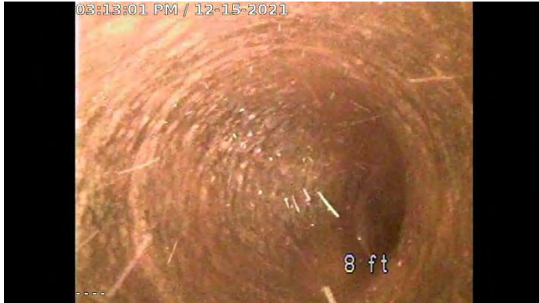
Photo from Drain Inlet #1 After Clearing
