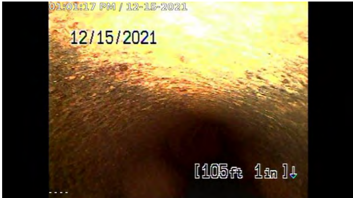
Photo from Drain #2 ( No Defects Observed)
